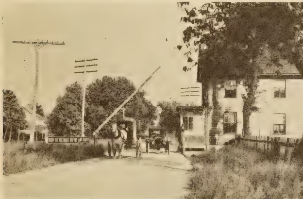
A NEW JERSEY TOLLGATE IN 1911
